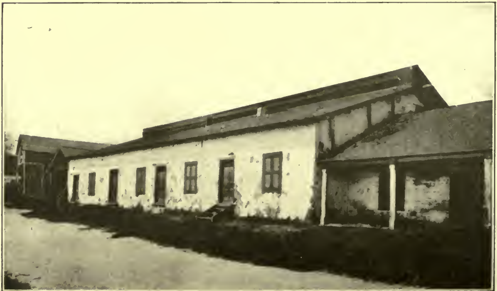
FIRST THEATER BUILDING IN CALIFORNIA —A type of the ancient adobe structure in old Monterey—It is said that the famous Jenny Lind on her first tour to the Pacific Coast in the fifties sang in this structure
